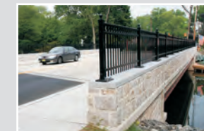
Springfield Avenue Bridge
