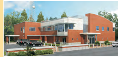
Bergen County Emergency 911/OEM Center
