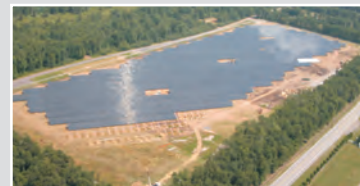
Pocono Raceway Park – Solar Field
